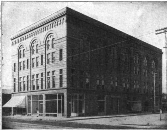
Marion County Telephone Company's Building, Marion, Ohio.
