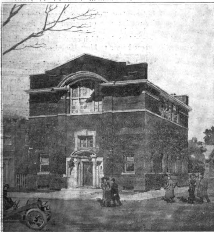
Branch Exchange Home Telephone Company of Detroit.
