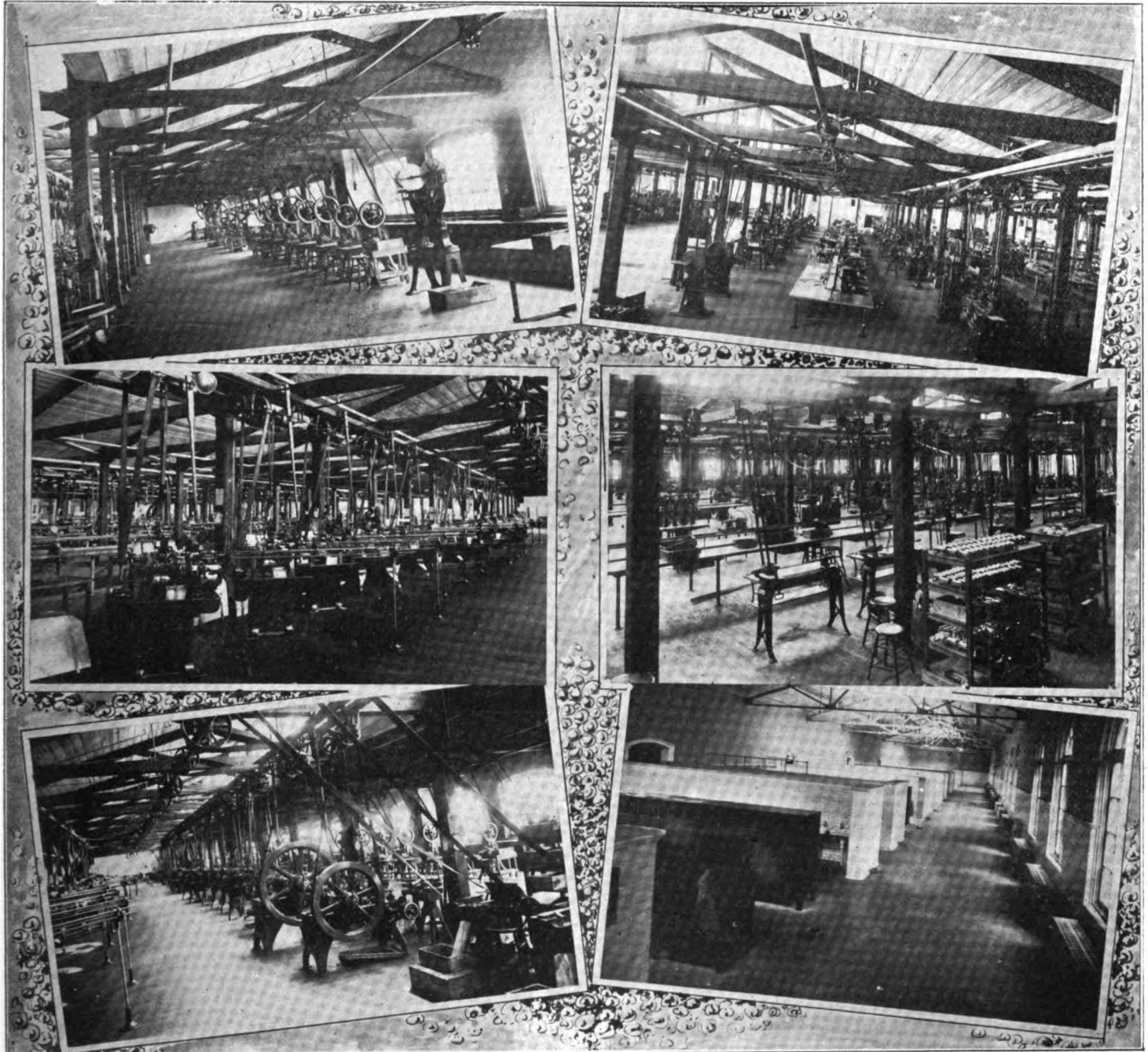
Figure 1—Press Room. Figure 2—Automatic Machine Room. Figure 3—Automatic Machine Room.
