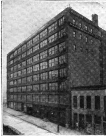
Western Telephone Manufacturing Company, Chicago.
