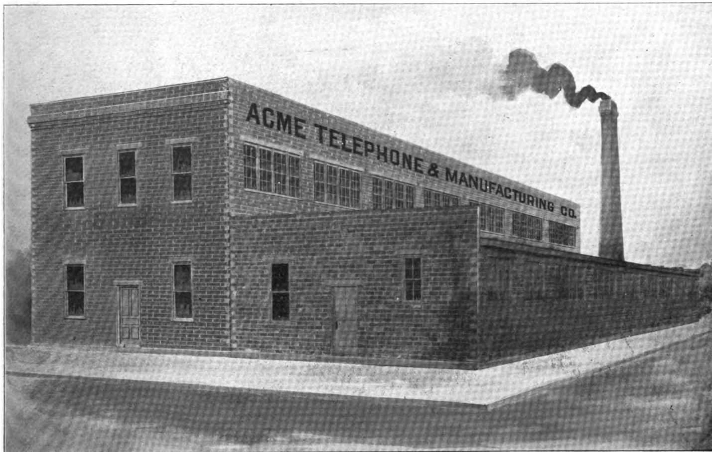
Factory of the Acme Telephone and Manufacturing Company. Albia, Iowa.
