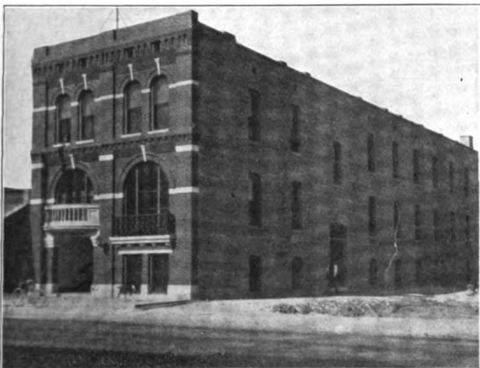
Figure 2—Southern Independent Telephone Company's Building.
