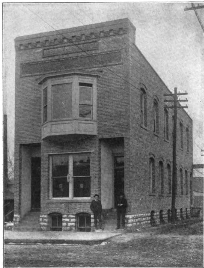
Building of the Albia Telephone Company, Albia, Iowa.
