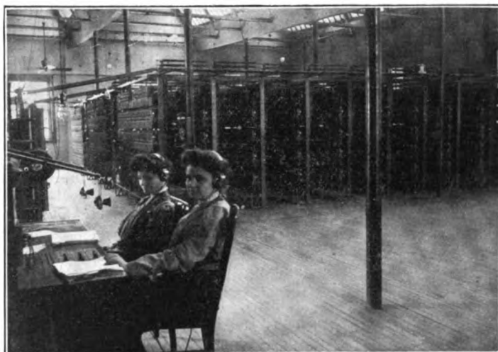
Automatic Switchboard of the Sioux City (Iowa) Telephone Company.
