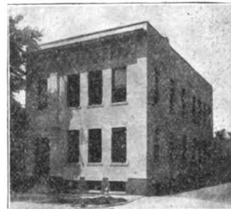
Wabash Valley Telephone Company, Paris
