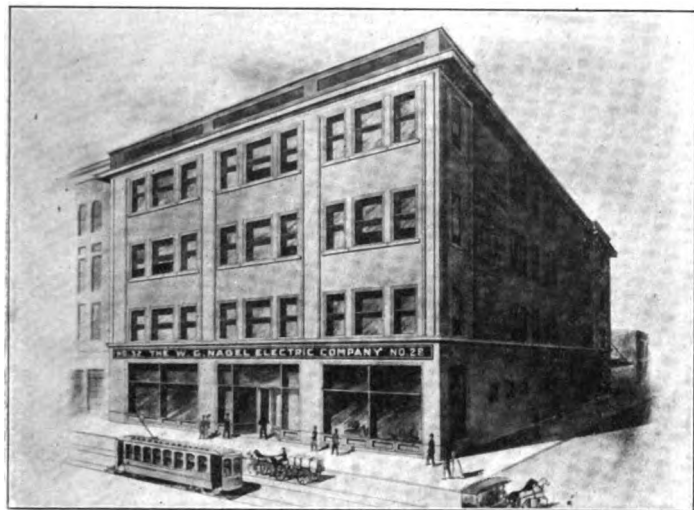
Factory W. G. Nagel Electric Company, Toledo, Ohio.
