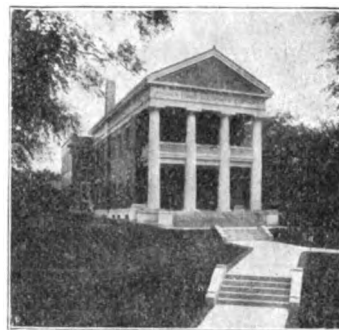
Home Telephone Company, Quincy.
