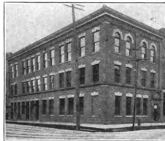
Independent Exchange Building, Ft. Wayne.
