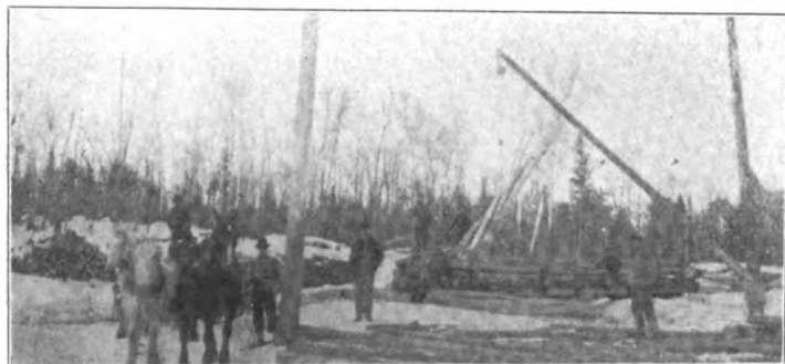
Method of Loading Poles.
