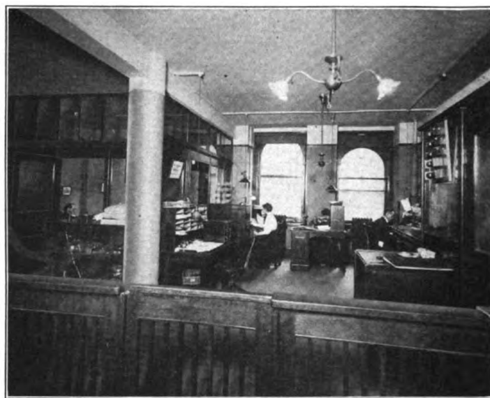
General Offices J. Allen Haines, Inc., Chicago.
