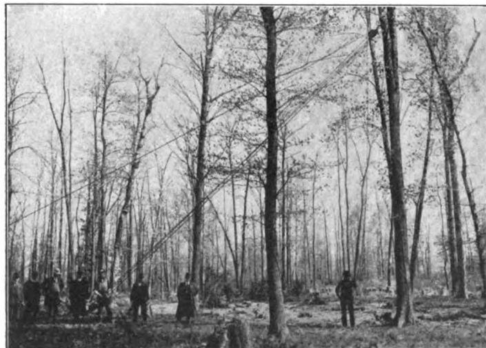
Wapak Anchor vs. a Twenty-Two Inch White Elm Tree Pulled Against Each Other by a Windlass Turned by Four Men.
