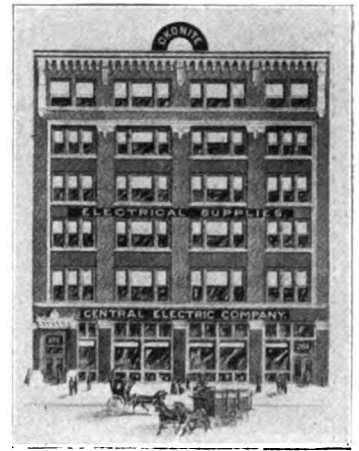
Central Electric Company, Chicago.
