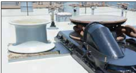
Capstan, wildcat and spurling pipe or "turtle-back" (black pipe anchor chain is going into)
