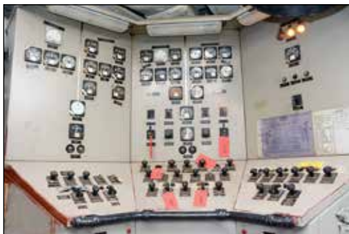
Electrical Control Panel
