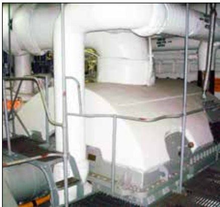
Low Pressure (LP) Turbine
