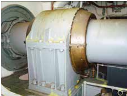
Shaft and Line Bearing
